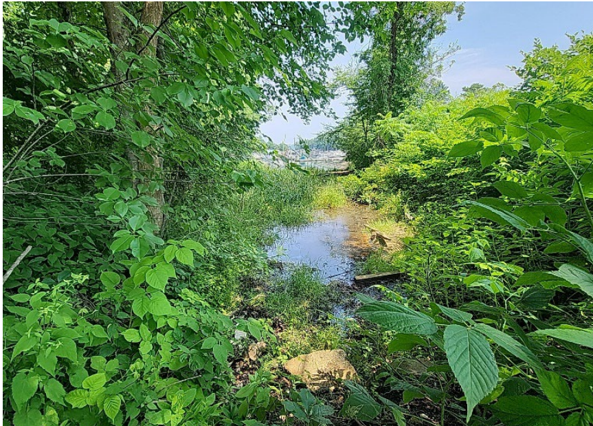
Photograph 9b: Looking east from storm drain pipe, note eroded bank along right, shows entire wetland remediation area; July 2024
